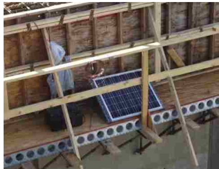
(a) Bent construction (thermocouples)
