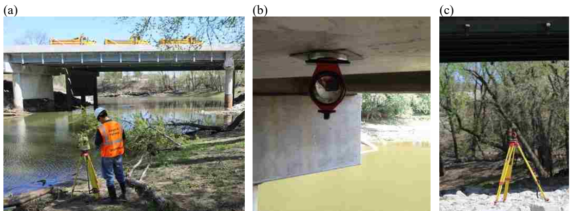
Figure 2. Automated total station.
