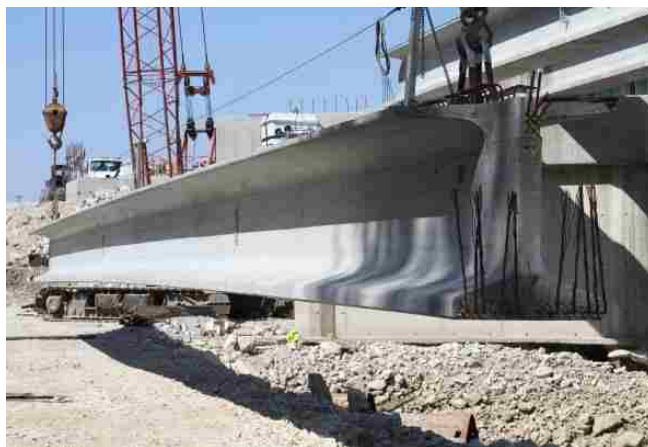
Figure 13. Girders erection.
