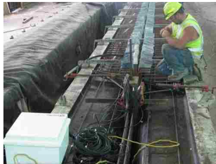
(b) Girders fabrication (VWSGs)
